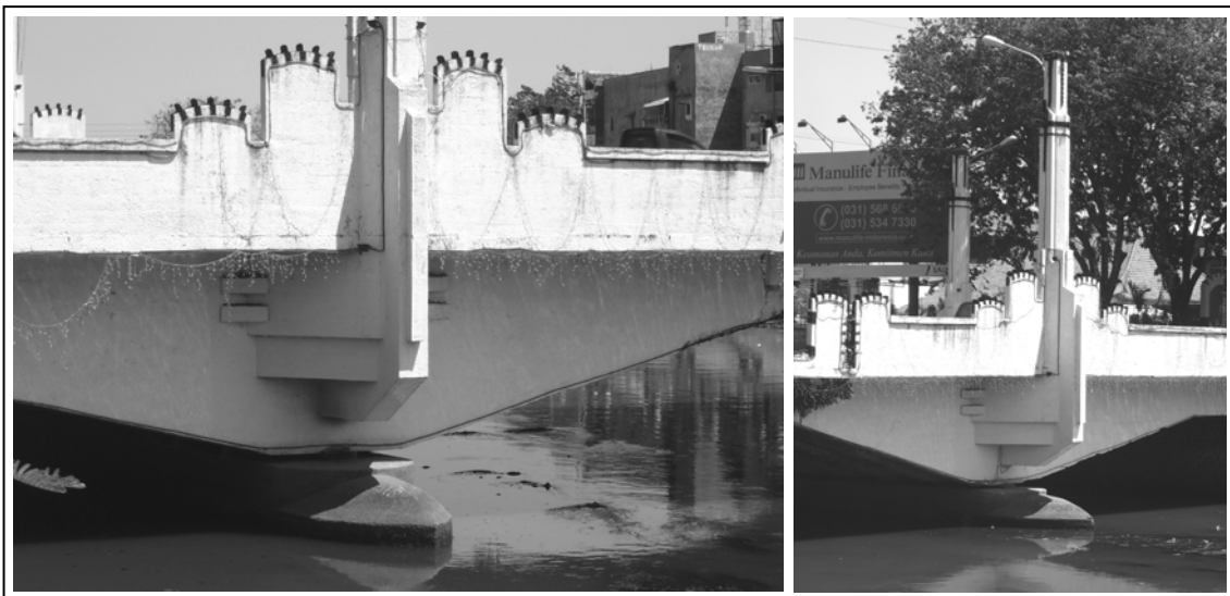
Fig.3.10.9. Gubeng Bridge: detail of the middle pillar.
