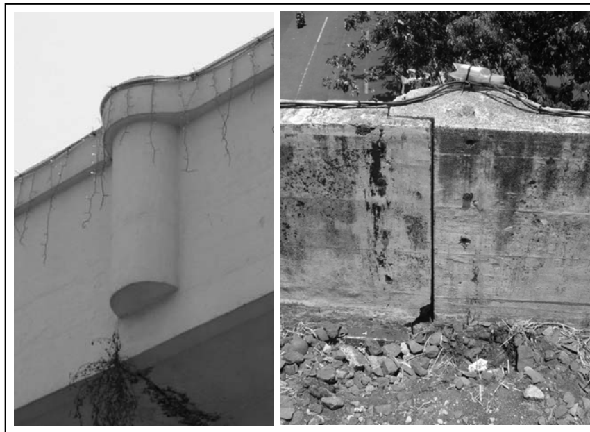
Fig.3.12.12. Pasar Besar Railway Viaduct: dilation joint
