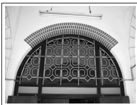
Fig.3.13.4. Old ASNI Building: arch with iron lattice work.
